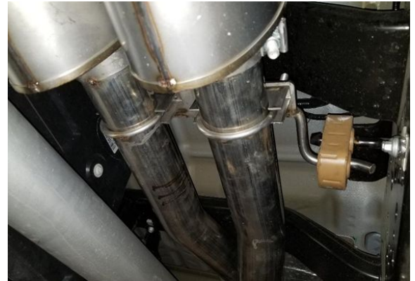
Detail 14: Inlet pipes to mufflers
