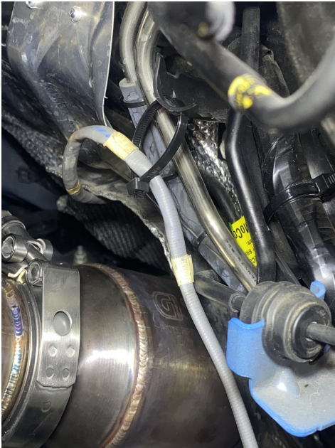
Detail 2: Bank 2 O2 sensor secured to the firewall using a zip tie to avoid contact with the cat.
