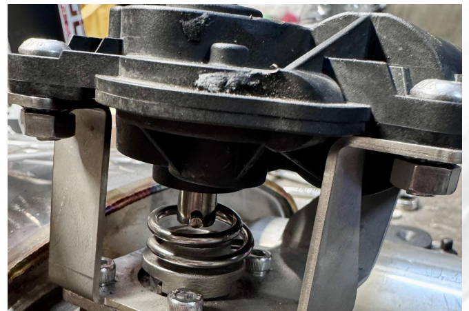
Detail 6: Valve motor mounted with spring and mounting screws.
