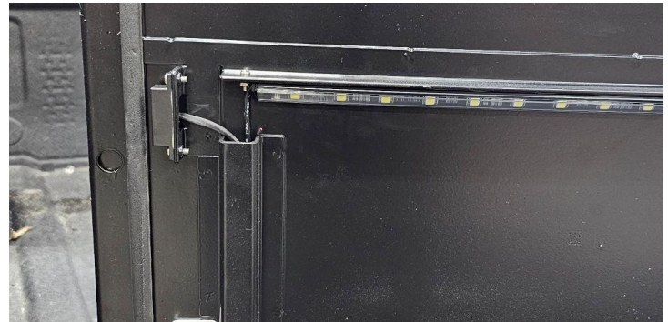
Detail B4: Left side light and magnetic latch installed
